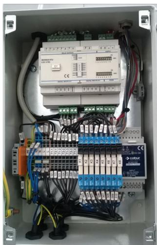
It is used to simplify the wiring harness in the plants with a large number of installed burners.
