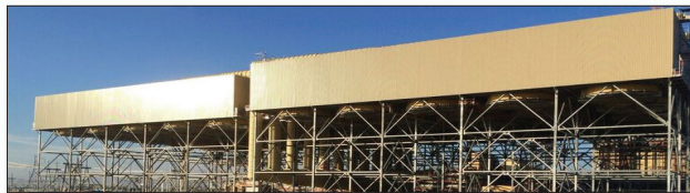
Butterfly arrangement to reduce overall height
