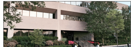
EVAPCO Dry Cooling, Bridgewater, New Jersey
