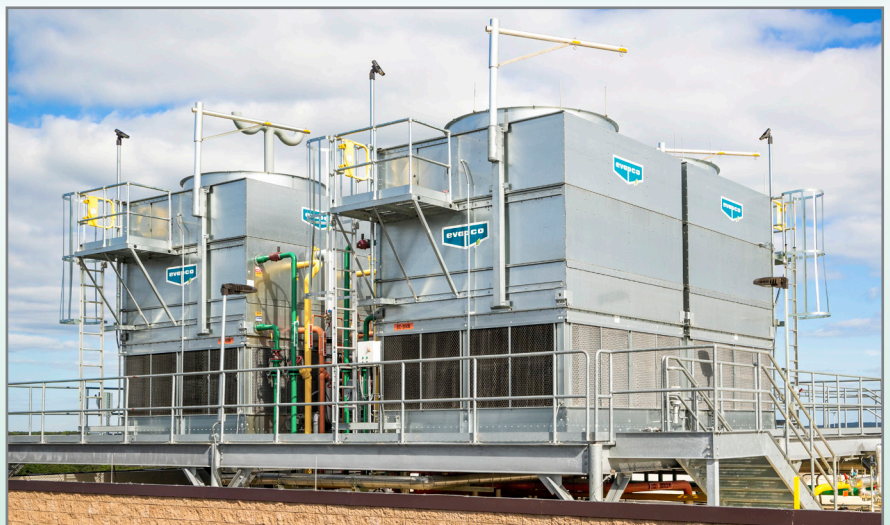
ATC-E Evaporative Condensers with external service platform.
