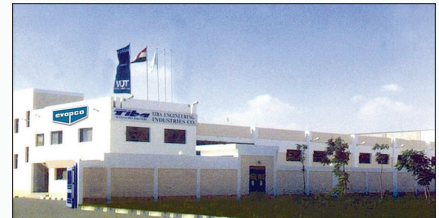
Evap Egypt Engineering Industries Co., Cairo, Egypt
