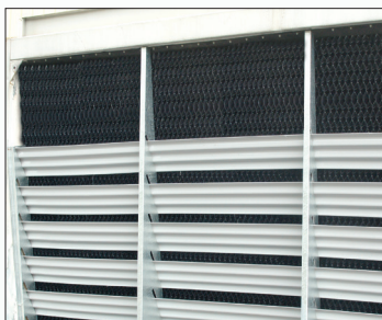
Improve thermal performance with high efficiency fill
