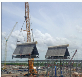
Modularization for efficient installations
