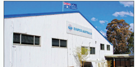
EVAPCO Australia (Pty.) Ltd., Riverstone, NSW Australia
