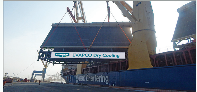
250-ton double fan module transportation
