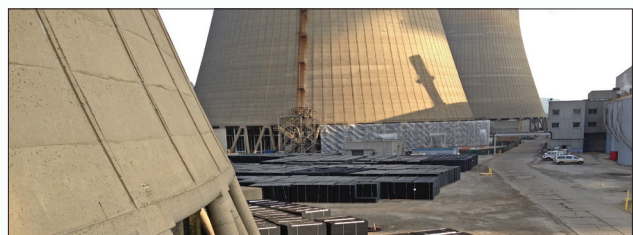
Major projects/Natural draft refurbishments
