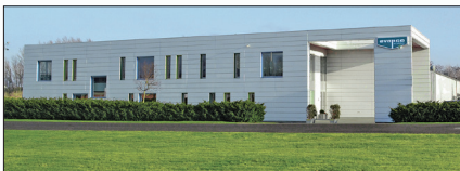
EVAPCO Air Solutions, Aabybro, Denmark
