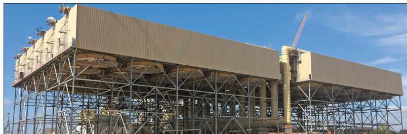
A strong focus on minimizing costs for traditional construction
