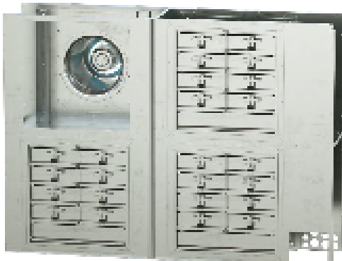
Figure 21: Backdraft Dampers
