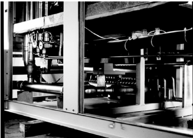
Figure 6: Economizer Piping
