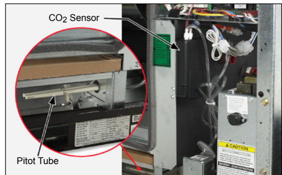
Figure 40: CO2 Sensor For Demand Control Ventilation
