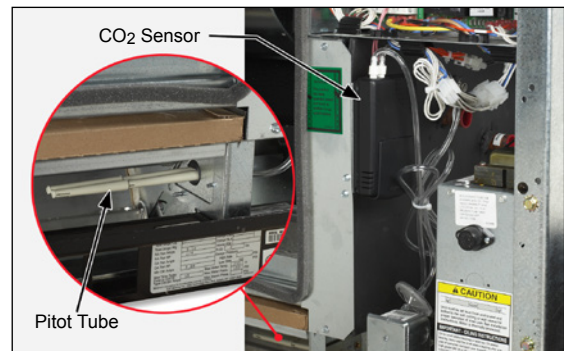
Figure 62: CO2 Sensor For Demand Control Ventilation
