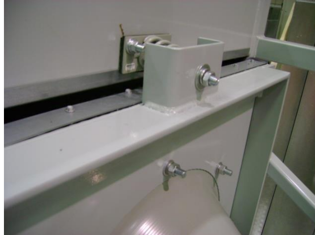
Thrust Restraint Spring
